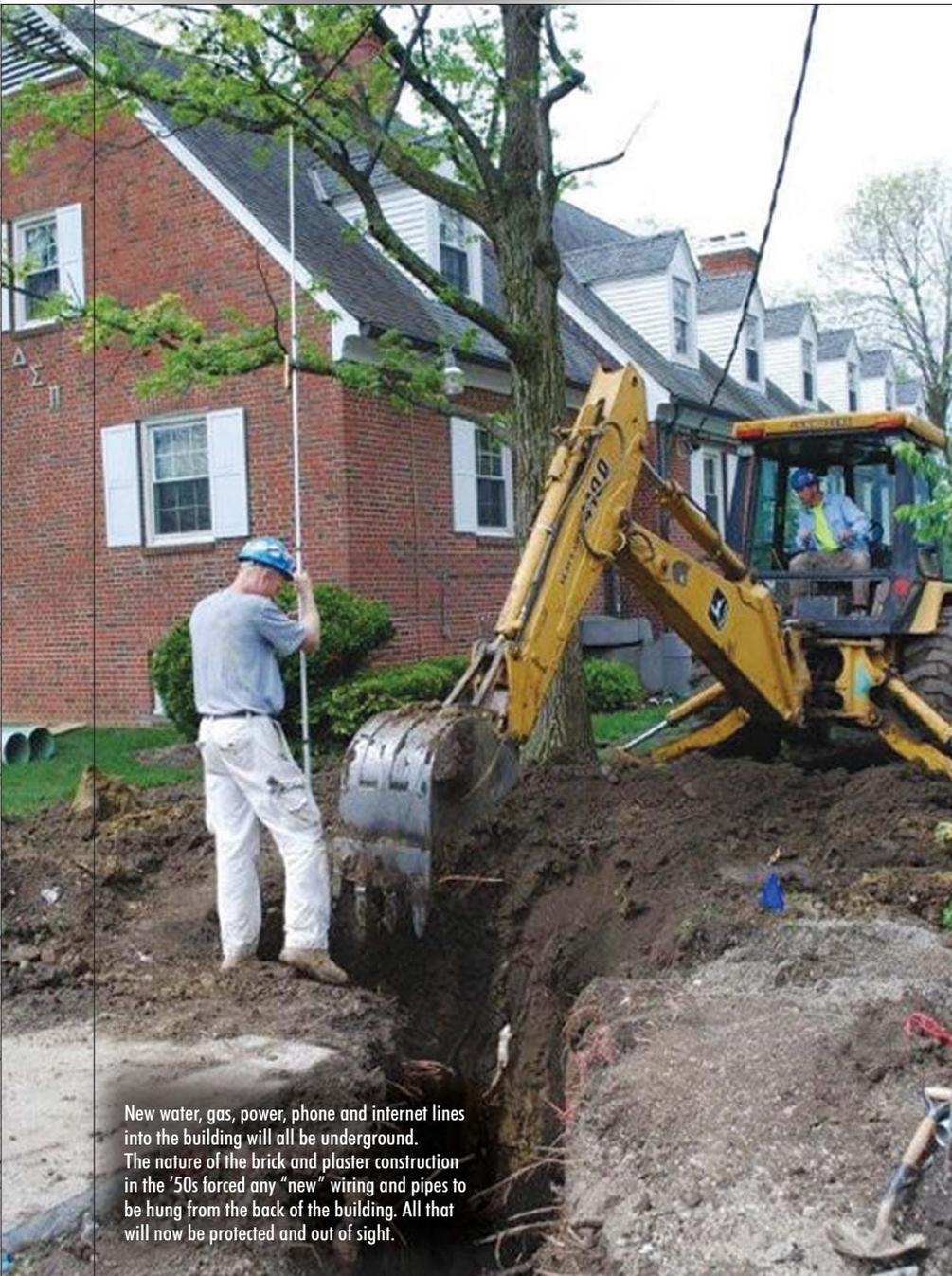
New water, gas, power, phone and internet lines into the building will all be underground. The nature of the brick and plaster construction in the '50s forced any "new" wiring and pipes to be hung from the back of the building. All that will now be protected and out of sight.
