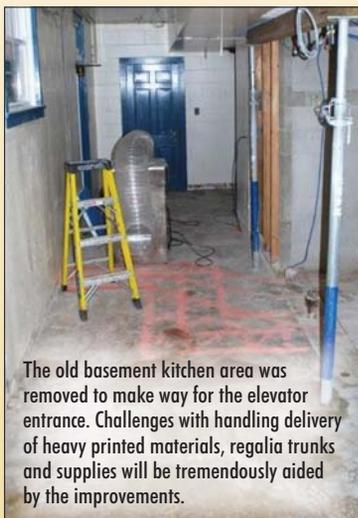
The old basement kitchen area was removed to make way for the elevator entrance. Challenges with handling delivery of heavy printed materials, regalia trunks and supplies will be tremendously aided by the improvements.
