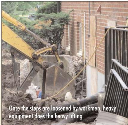
Once the steps are loosened by workmen, heavy equipment does the heavy lifting.
