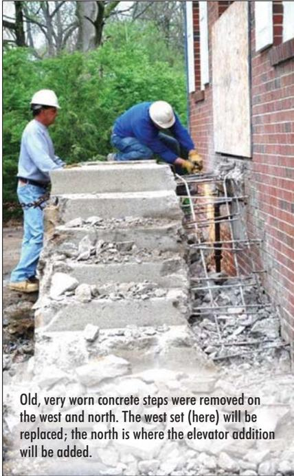
Old, very worn concrete steps were removed on the west and north. The west set (here) will be replaced; the north is where the elevator addition will be added.
