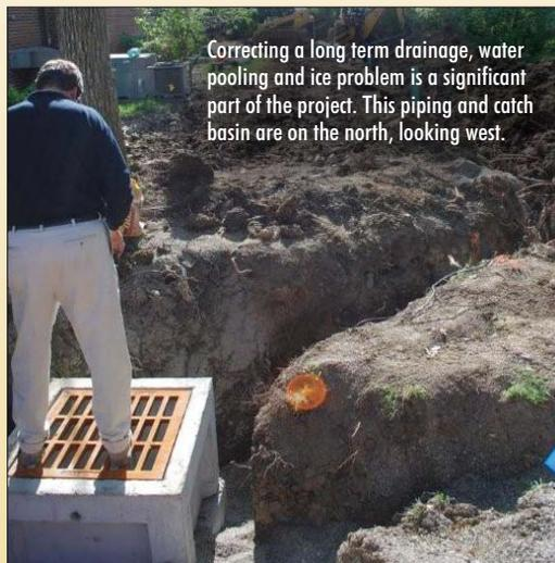
Correcting a long term drainage, water pooling and ice problem is a significant part of the project. This piping and catch basin are on the north, looking west.
