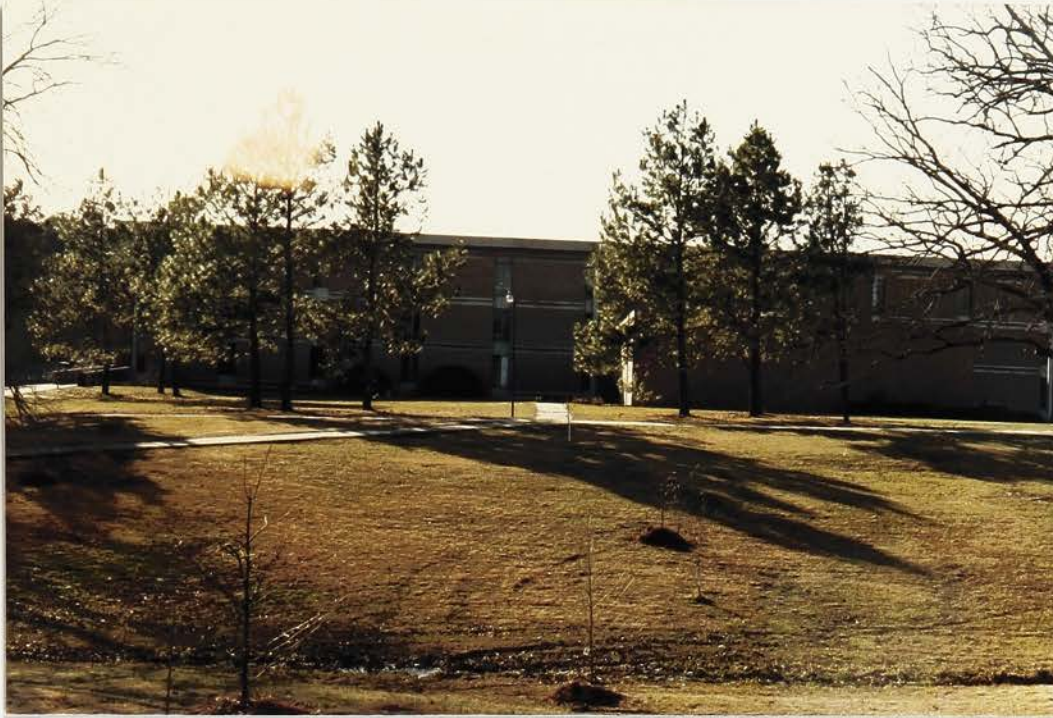
Lurleen Burns Wallace Hall provides instructional facilities for chemistry, physics, English, history, the social sciences, business and industrial education. This building also contains a small auditorium.
